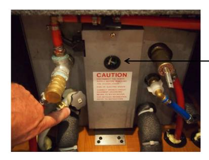
Try to remember not to engage the lighted water heater switch while the engine block is still; by doing this, you take the risk of tripping the reset breaker on the thermostat of the water heater. The <u>reset button</u> is located on the water heater unit, accessible through the small hole on the front panel of the water heater shown in the above picture.
