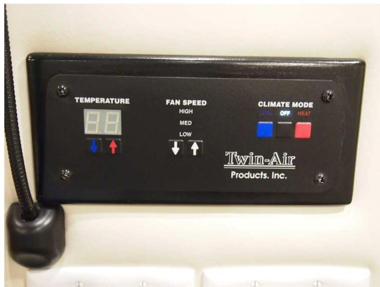
The fan control for the secondary auxiliary heater is located here on the control panel, as shown below.
