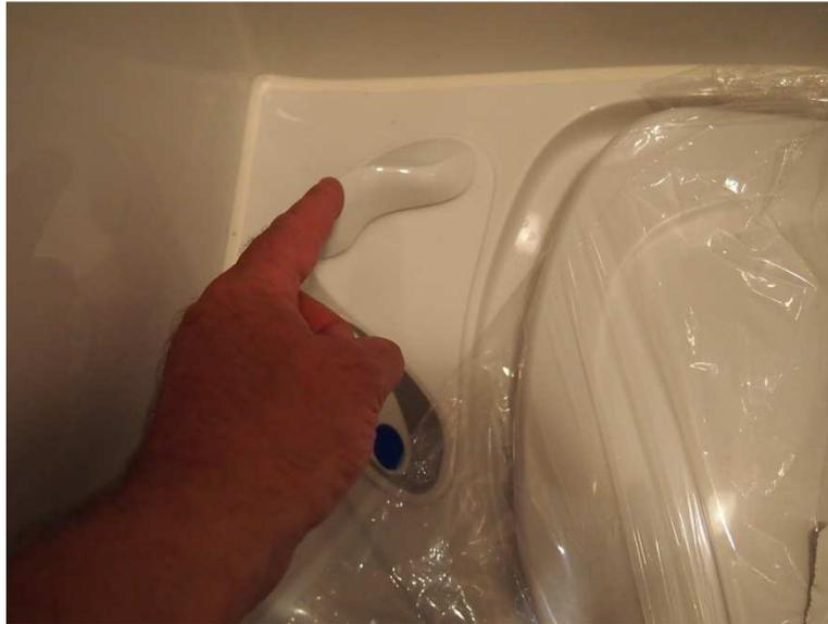
This button, shown below, is used to fill the toilet bowl with clean flush water.
