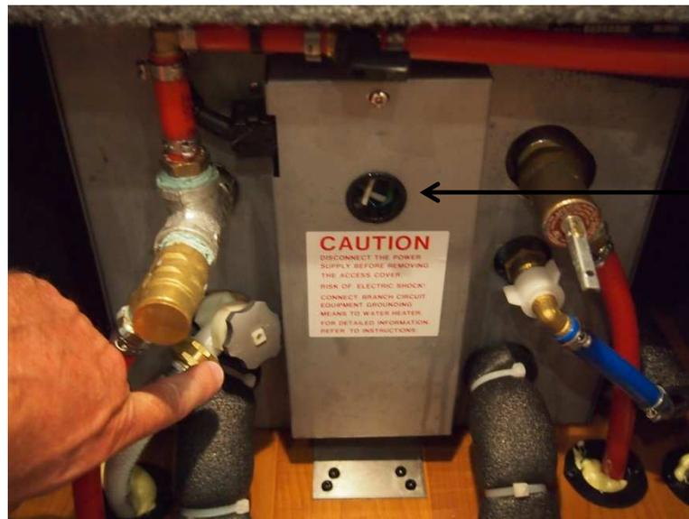
Try to remember not to engage the lighted water heater switch while the engine block is still hot; by doing this, you take the risk of tripping the reset breaker on the thermostat of the water heater. The reset button is located on the water heater unit, accessible through the small hole on the front panel of the water heater shown in the above picture.
